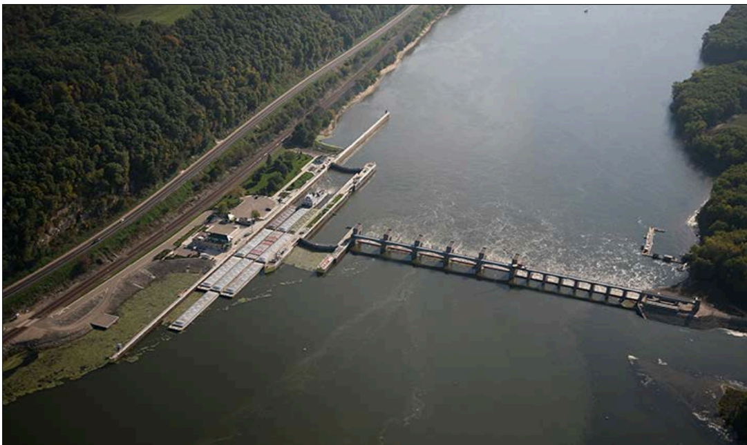
Figure 3.2(b). Lock and Dam 9 on the Mississippi River near Lynxville, Wisconsin. A similar structure would likely be required on the Missouri River for diversion rates in excess of 6,000 cfs.
